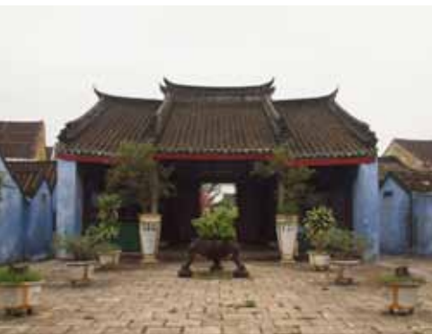
One of the many well-preserved clan houses in Hoi An
