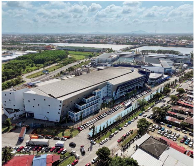
ST Muar's facilities and operations have expanded over the last five decades
