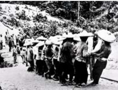
Coolies hauling a boiler uphill, 1911.
