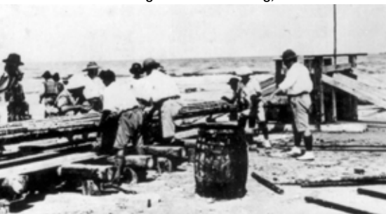
Launching a sealine in Lutong, 1921.
