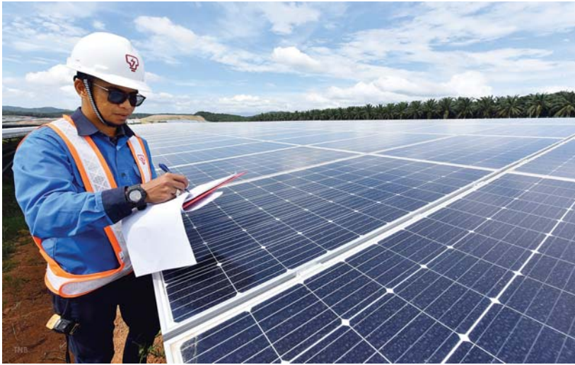
A Tenaga employee on site at the LSS Bukit Selambau
